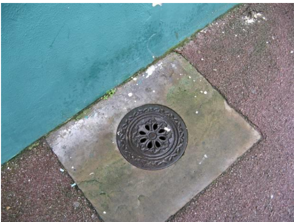
Cast iron coal hole in Grotto Road
