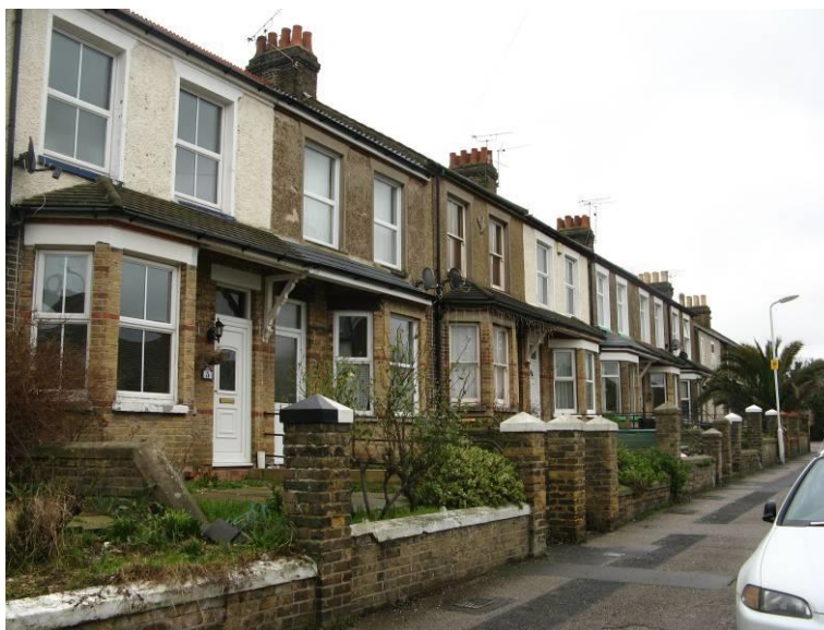
Houses in Grotto Gardens
